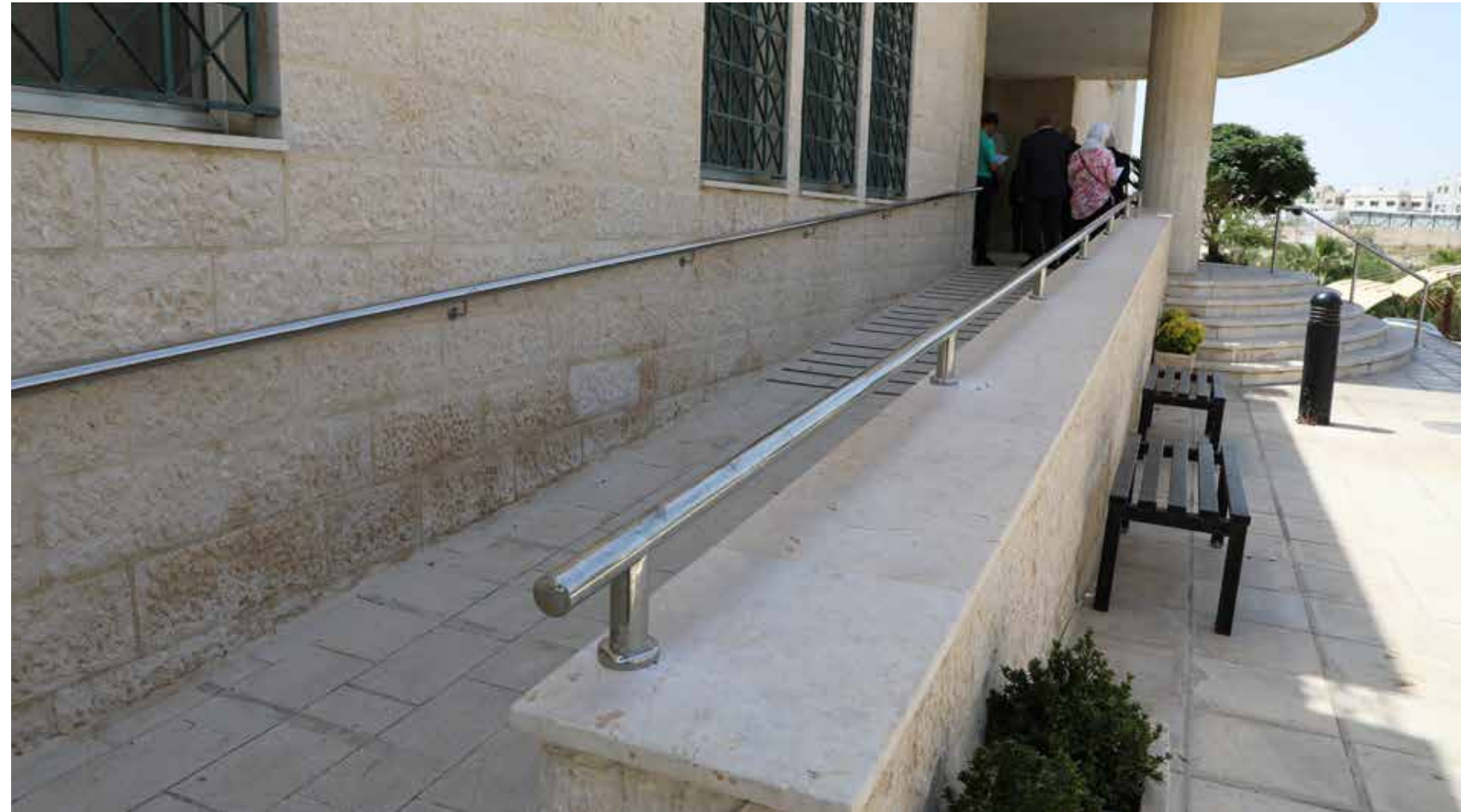
Construction of ramps that meet the specifications of the Building Code Requirements for Persons with Disabilities.
