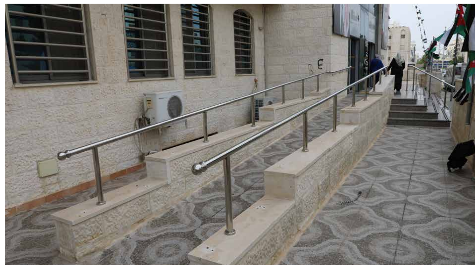
Installation of ramps that comply with the Building Code Requirements for Persons with Disabilities.
