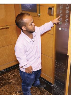
Accessible Elevators: ifts designed with sufficient space for wheelchair manoeuvring. They feature a low level control panel with Braille labelled, illuminated buttons; an audio system to announce floor levels; wide doors; generous internal dimensions; horizontal side supports; an interior mirror; and a fold away seat for persons using mobility aids.
